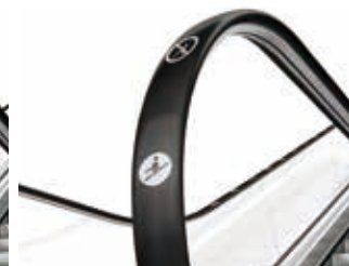
Safety signage handrail
